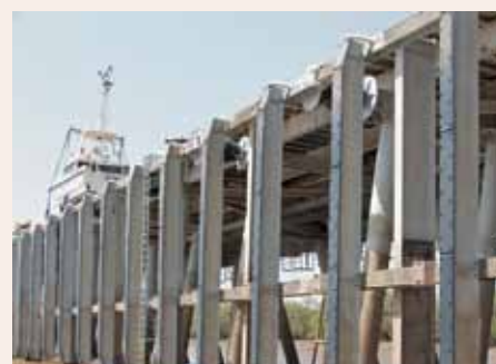
Sturdy stuff . . . after-shots of the Port of Wyndham's jetty piles.
