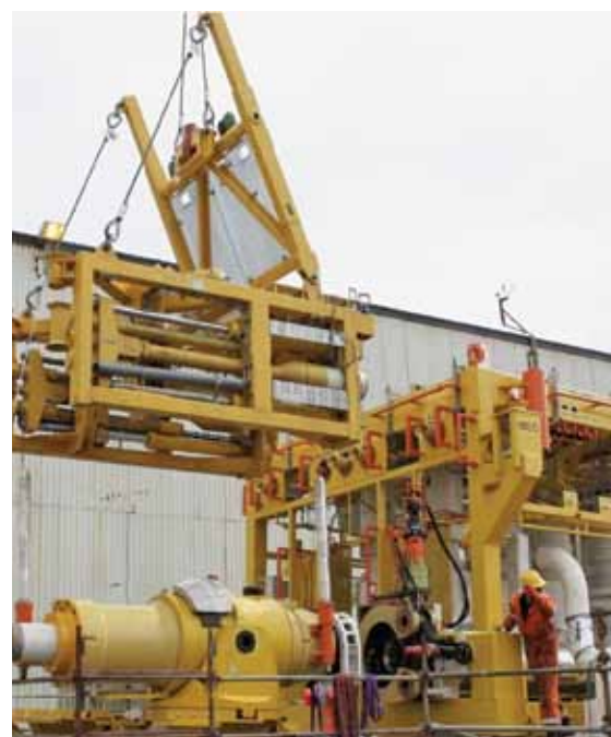
A well head tree being assembled. Photo: FMC Technologies.
