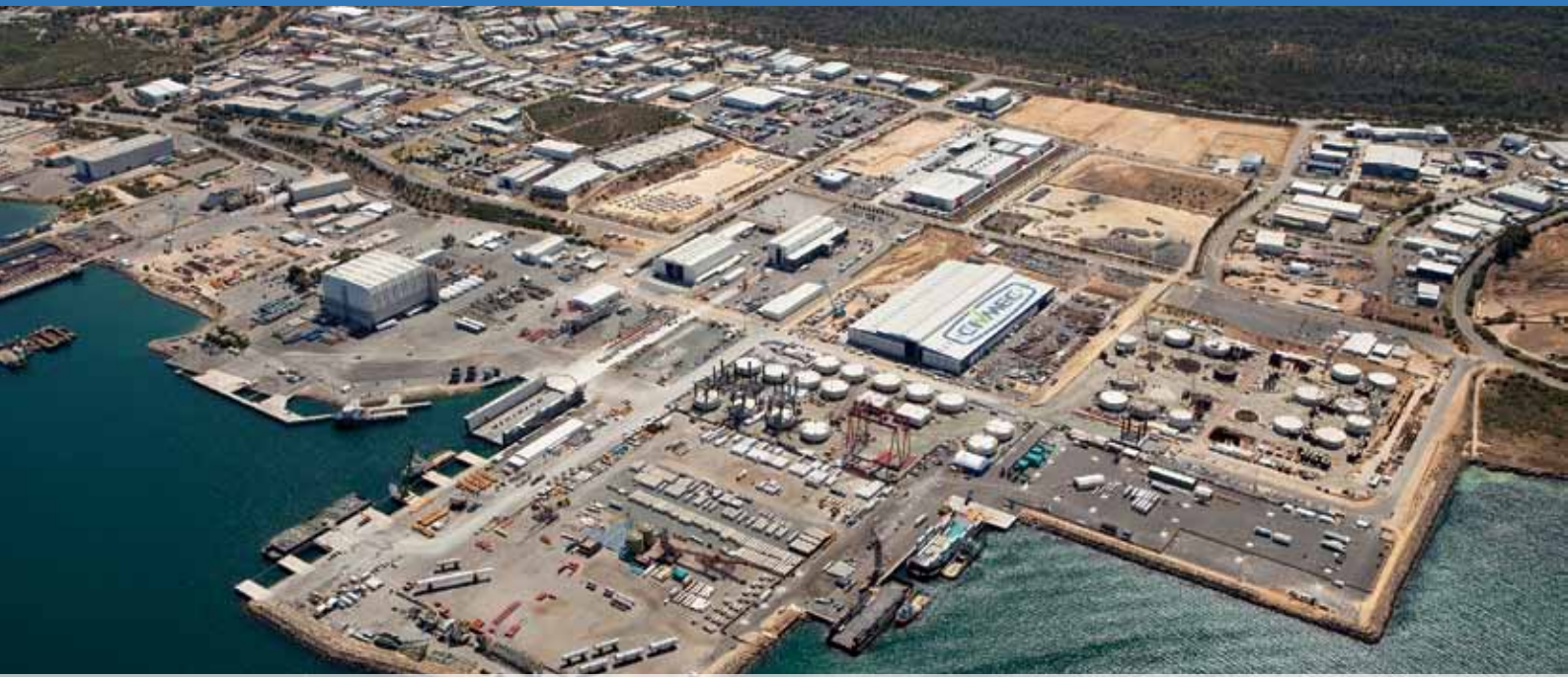
The 20,000 square metre Matrix facility at the AMC, Henderson. Photo: Matrix.
