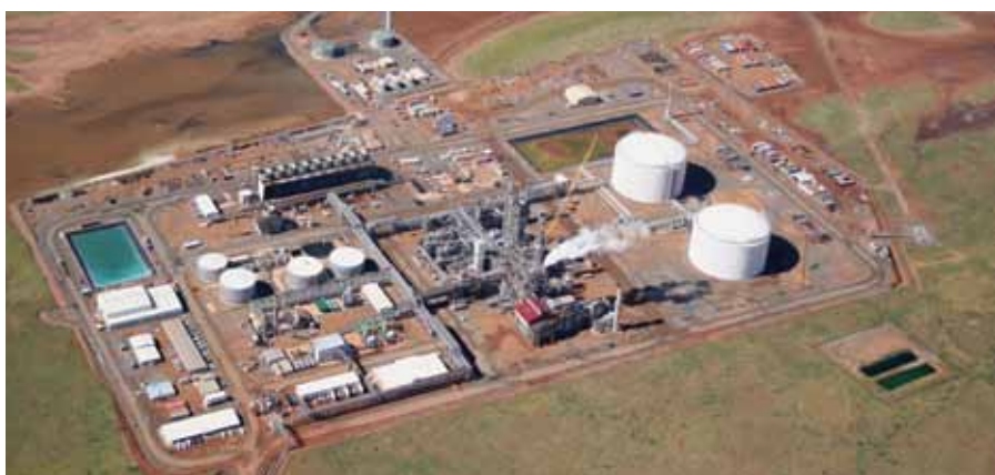
Aerial shot of the Burrup liquid ammonia plant.
