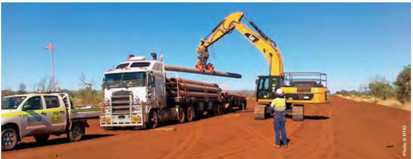
The Deckhand® being used for the first time in Australia to construct the West Angelas pipeline
