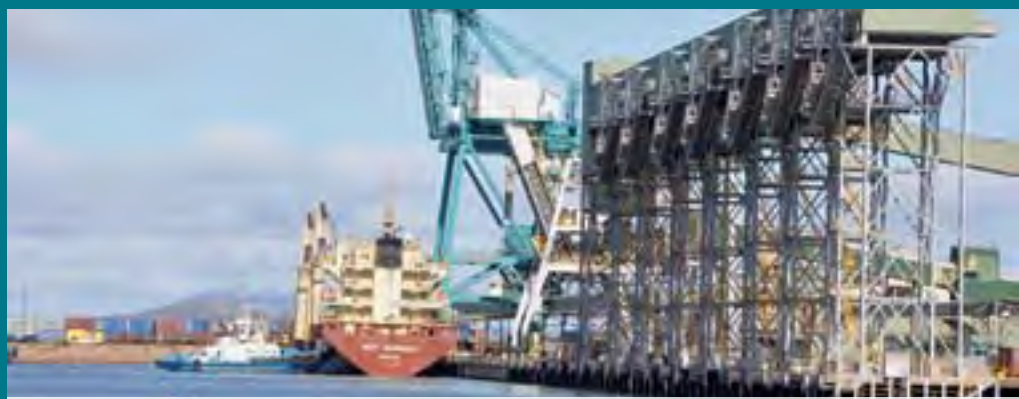
The Esperance Port is set for a $200 million upgrade.
