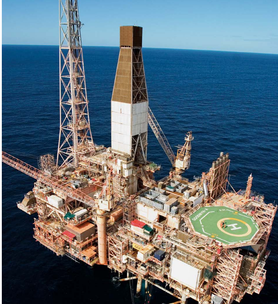
Woodside's Goodwyn A gas platform, North West Shelf Project, Western Australia, received a 3D printed part in 2016. In collaboration with Monash University, the part was on its way to site within three days. Photo: Woodside Energy
