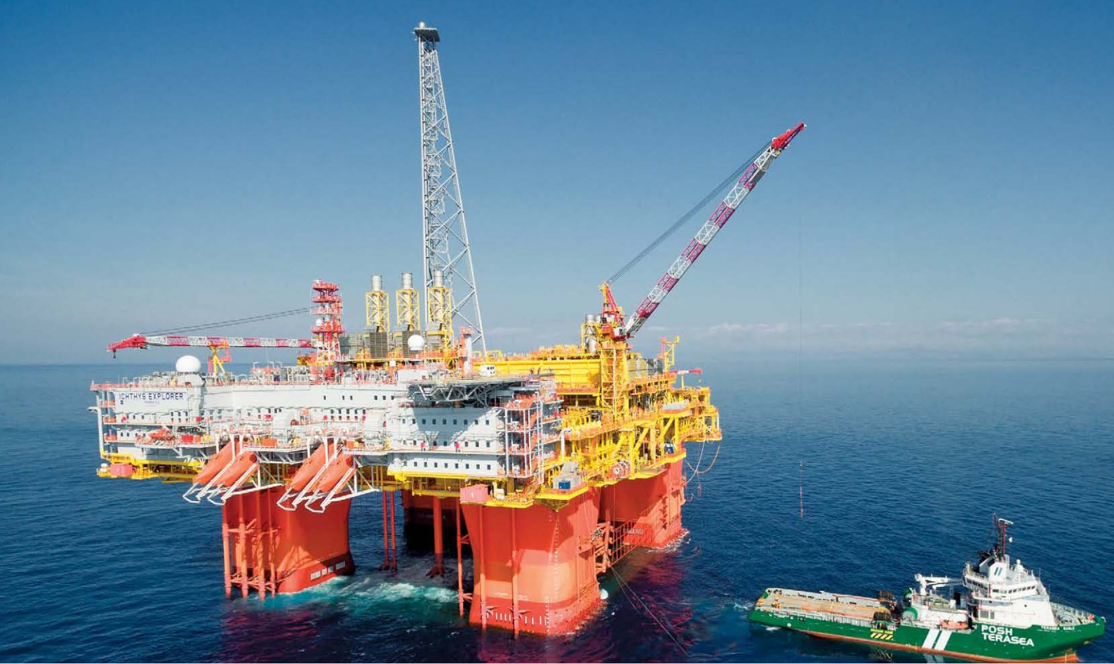
INPEX-operated Ichthys LNG Project's central processing facility (CPF) "Ichthys Explorer". Photo: INPEX
