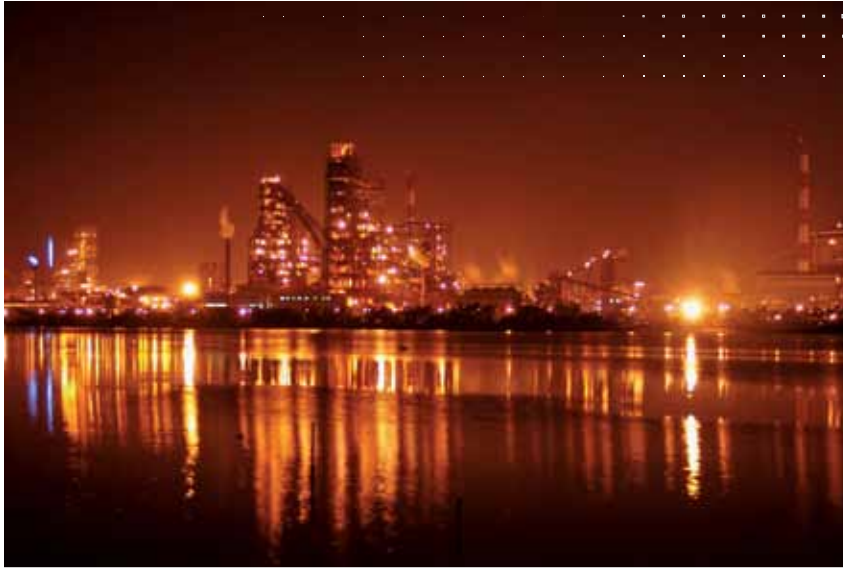
POSCO steelworks in South Korea. Photo: POSCO.
