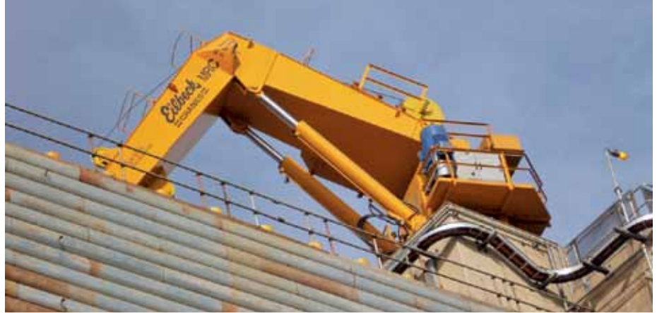
Etschmann Engineering was fined A$16,000 following the structural collapse of an 80-tonne crane during test loading in April 2013.
