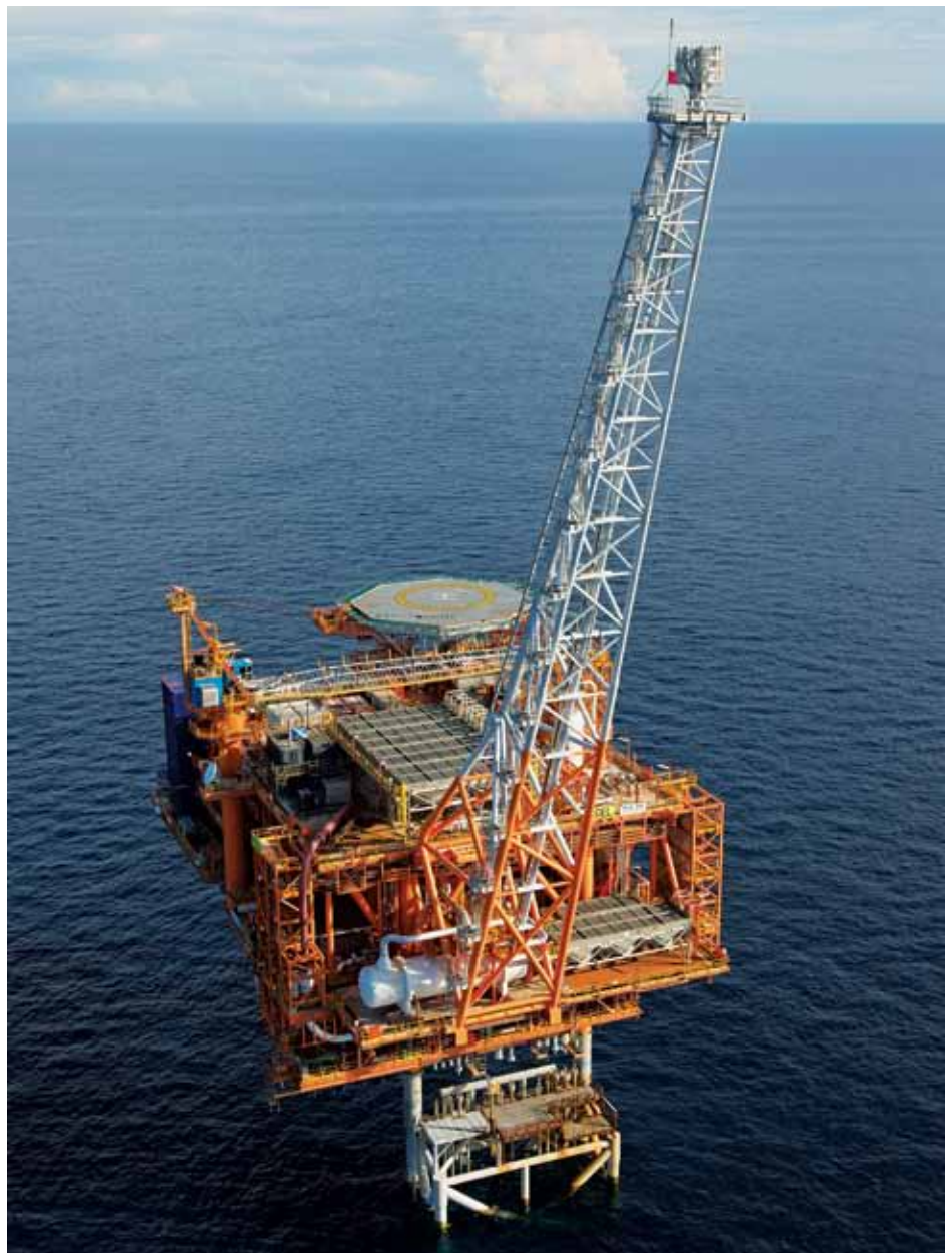
The Angel platform, an offshore gas production facility that is part of the North West Shelf Joint Venture. Photo: Woodside Energy Ltd.
