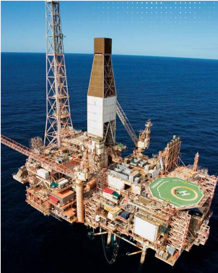
Goodwyn A gas platform, North West Shelf Project, Western Australia. Photo: Woodside Energy Ltd
