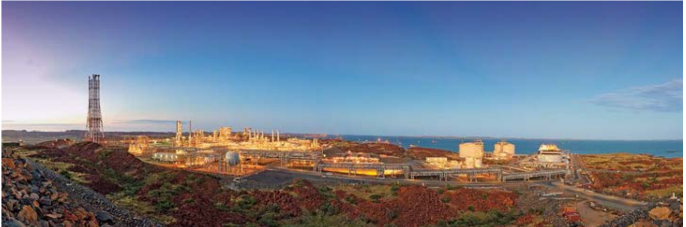
Woodside's Pluto LNG onshore gas plant in Western Australia's North West. Photo: Woodside Energy Ltd
