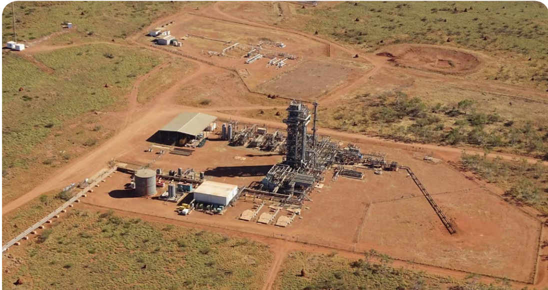
Aerial view of the Tubridgi gas well site.
