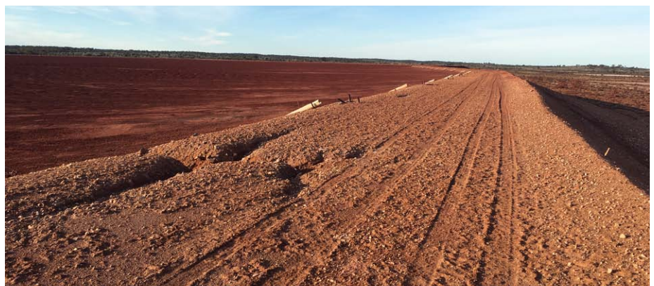
Internal road at the Bulong tailing storage facility.
