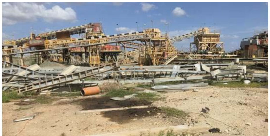
Ellendale Diamond mine processing facility.
