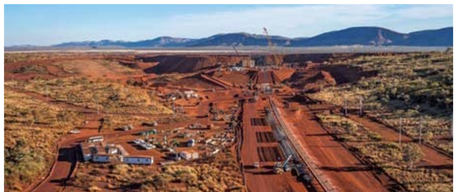
Rio Tinto's $468 million Silvergrass iron ore mine in Western Australia's Pilbara region. Photo: Rio Tinto
