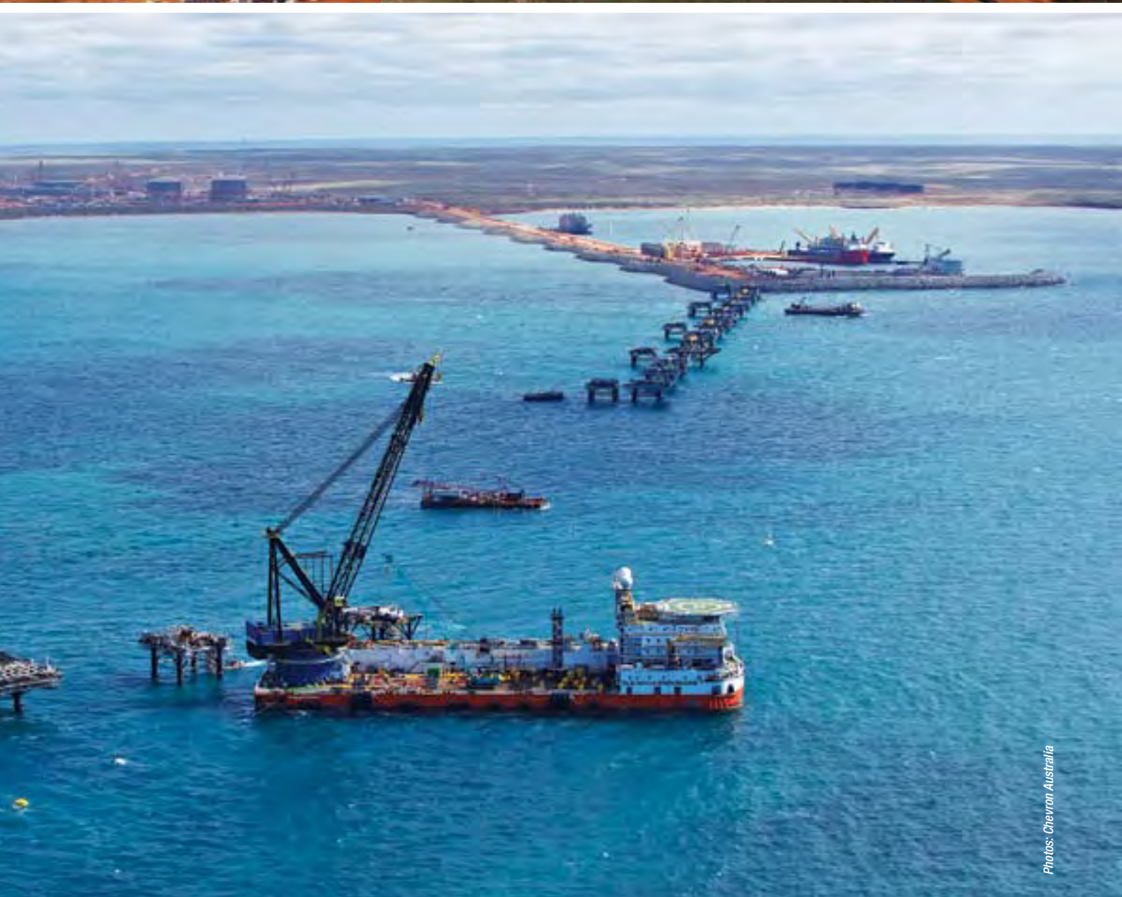
Top left: Foundations have been poured for all five gas turbine generators, which will provide standalone electrical power generation for the LNG plant and associated facilities. Top right: Construction on the Gorgon Operations Centre is progressing at the Permanent Operations Facility site. Above: Work continues on the 2.1km LNG jetty with 24 caissons in place at the beginning of August. Installation of the jetty roadways is underway.
