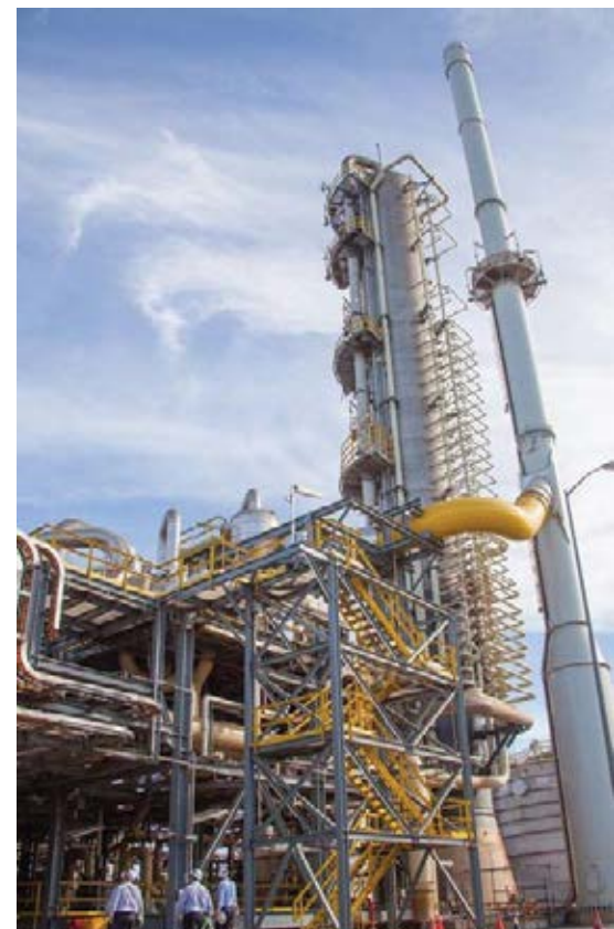
The Yara Pilbara Nitrates plant. Photo: Yara.
