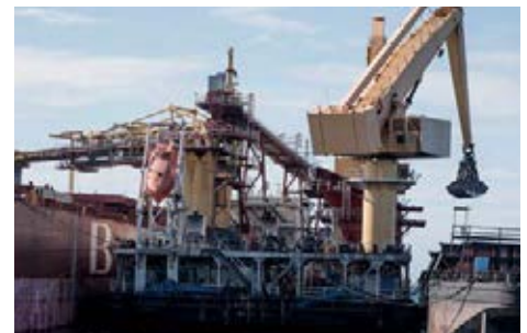
The bulk export port developed for the Sino Iron project. Photo: CITIC Pacific.
