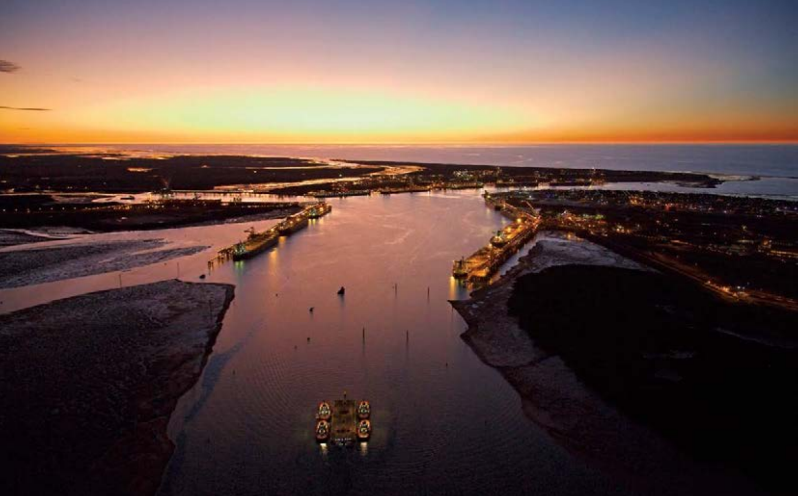
Aerial view of the port of Port Hedland, which now has the largest throughput of Australia's ports. Photo: Pilbara Ports Authority.
