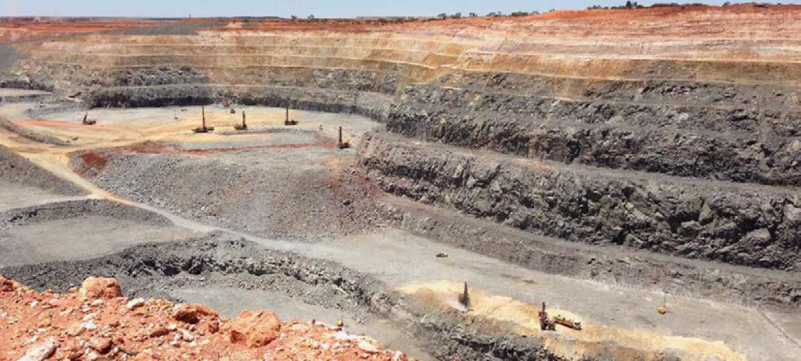
The Tropicana Gold Mine was one of the first Lead Agency Projects to start production.
