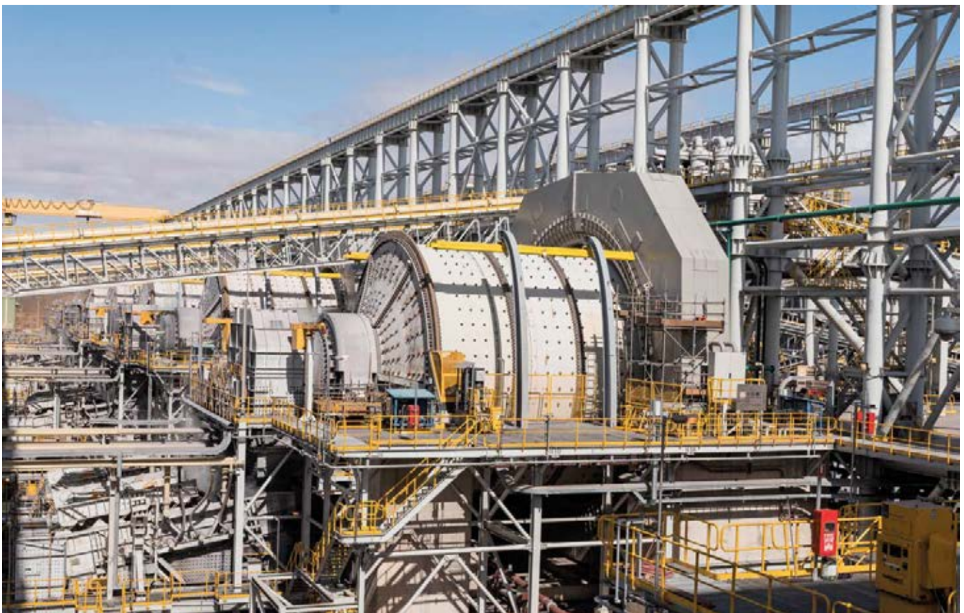
More than 4000 people were involved in building the Sino Iron project. Photo: CITIC Pacific.
