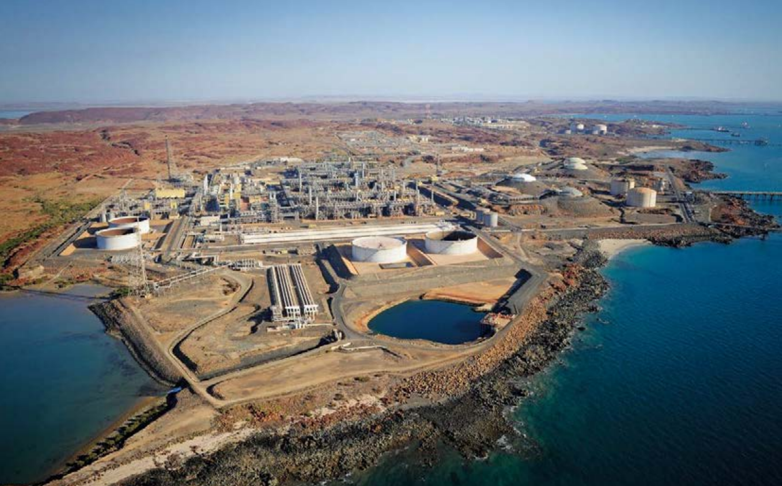
Karratha Gas Plant, North West Shelf Project, Western Australia. Photo: Woodside Energy Ltd.
