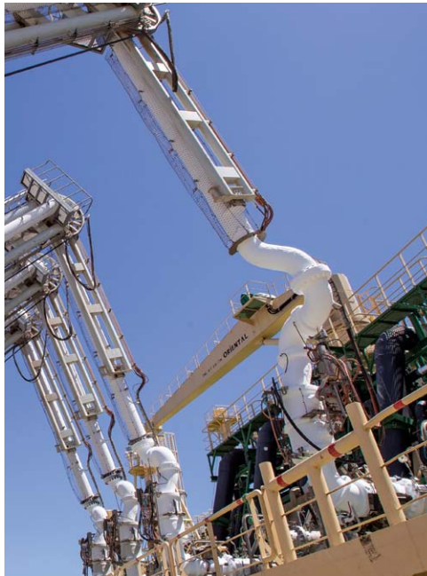
Loading arms transfer the first cargo of Wheatstone LNG to the Asia Venture. Photo: Chevron
