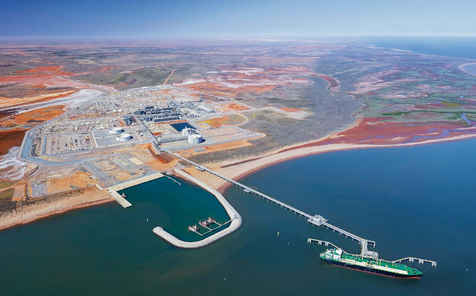
The first shipment of LNG set sail from the Chevron-operated Wheatstone Project in October. Photo: Chevron
